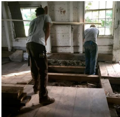
Photo left: Tucker Trapp and Adam Nelson carefully remove, mark and place floorboards off-side to expose floor joists and sleepers. Wentworth Brown Carriage Barn, August 20, 2020.
