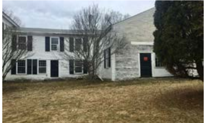
ca. 1790 small house and barn, south facing elevation
